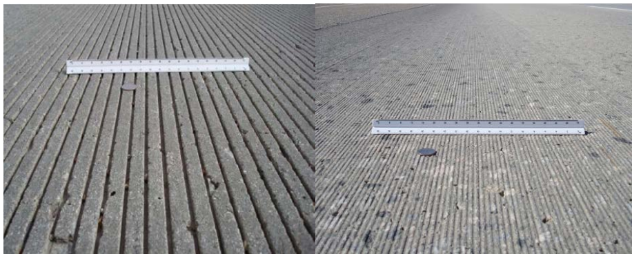
Figure 10. Grooved Surface (Left) and Diamond Ground Concrete Pavement Surface (Right).
