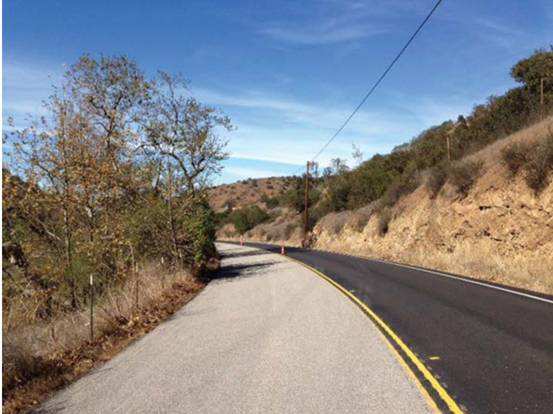
Figure 17. High-Friction Surface Treatment on a Horizontal Curve (53).
