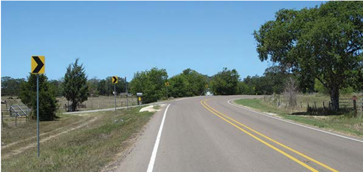
Figure 16. White Edgelines, Centerline RRPMS, and Chevrons on a Horizontal Curve (53).
