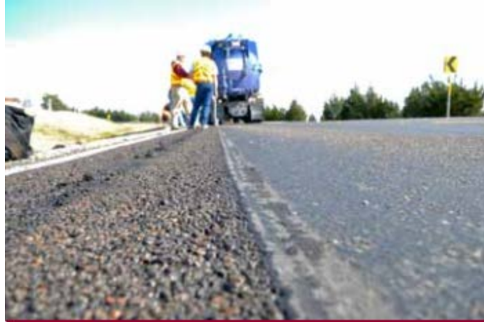
Figure 11. Effects of Water Blasting Test (32).
